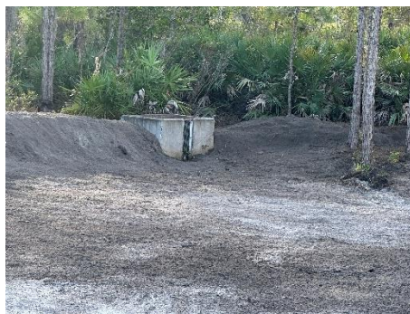
Walls and Overflow structure
