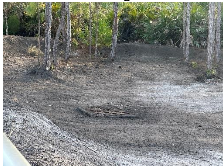
Remade with inlet grid
